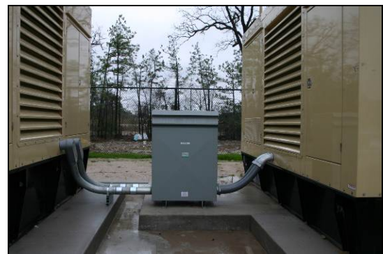
Photo of GenLink DPNL installation
