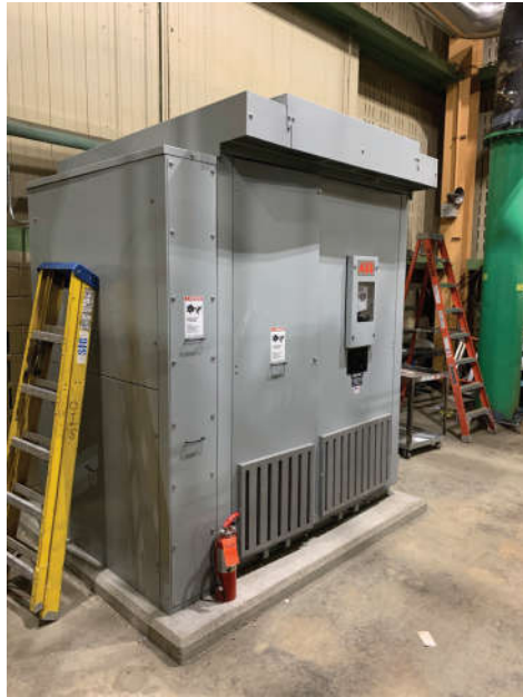
2.4kV-480V, 500kVA Cast-Coil Transformer
